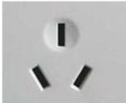
The standard wall plug in most households in China has a grounding pin and two power conducting pins in a V-shape:
