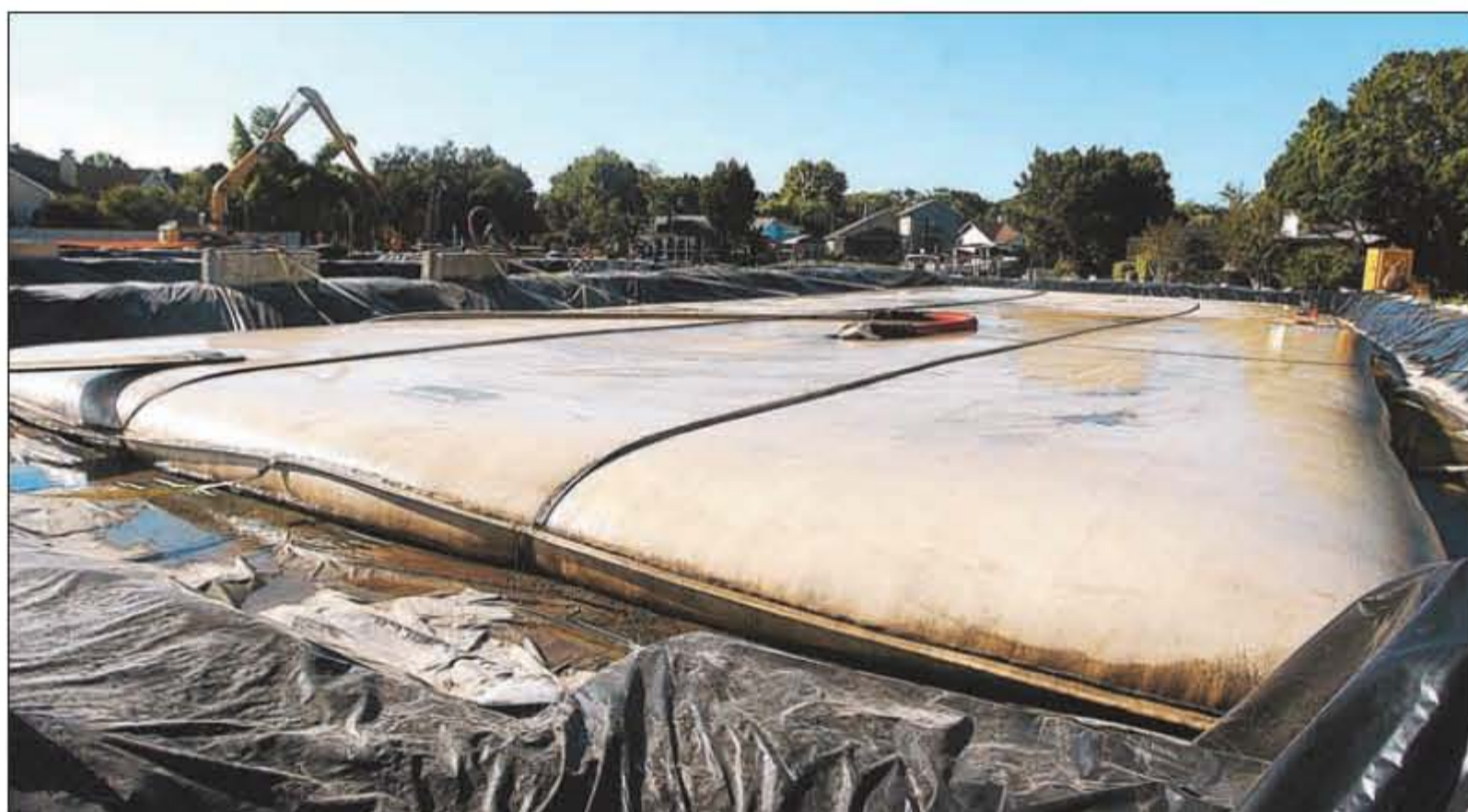
The large-scale operation that Save Crystal River has spearheaded has a land-based element where water and debris is filtered, separated and eventually returned to the environment.
