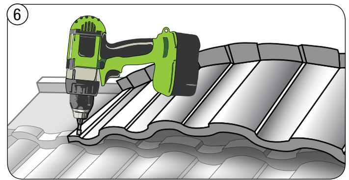
Then fasten at bottom far left corner. Panels are then pushed down to fit coursing properly.
