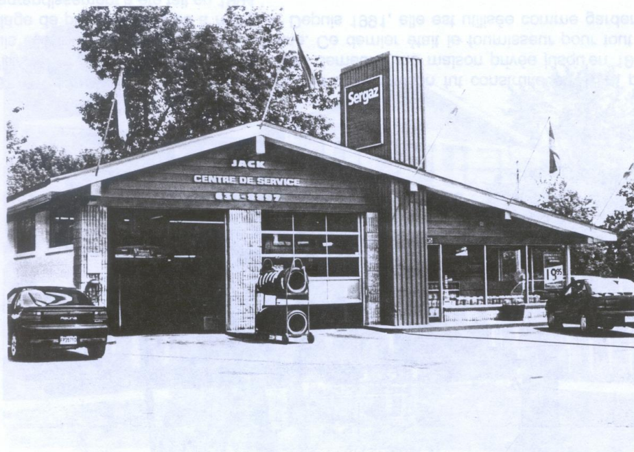
505 Lakeshore: The first garage in Dorval was built here in 1915 by Aldée Boyer, father of Roland and included a small hardware store. It was later run by Arthur Samson as an Esso station but burned down in 1960. Rebuilt as a Texaco station, it was run by Frank Richmond until his death in 1990 and is now a Sergaz station run by Jack Levy.
