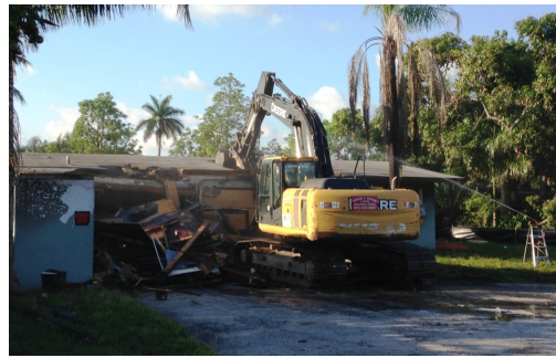
The demolition starts, right thru the roof
