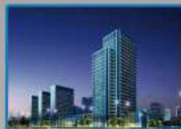
Networked Security: Building
