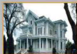
Access Control: House
