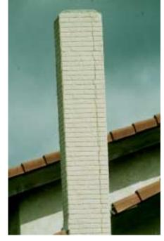
reinforcement. When the calcium chloride is mixed with moisture a reaction occurs and rust scale develops on the steel reinforcement. This reaction and expansion of the steel reinforcement causes fractures in the concrete. These cracks always start on the exterior surface first.
