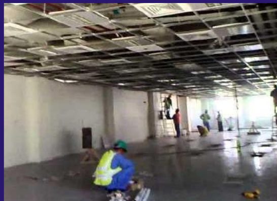
Ceiling works (Cables-fire protection-AC-lights)
