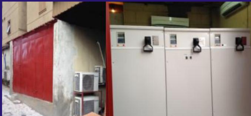
14. VICTORIA CROWN PLAZA HOTEL 1000 KVA 320 -450 VAC IN /400 VAC 50 HZ %1-5 OUTPUT VOLTAGE STABILISER DESIGN , SUPPLY, ROOM CONSTRUCTION , CABLING WITH 1X500 MM ARMoured CABLE, 1250 AMPER SCHNEIDER MCCB BUILT IN PANEL , BREAKER AND COMMISSIONING
