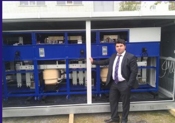
8.TURKMENISTAN 1600 KVA OUTDOOR AIR COOLED VOLTAGE STABILISER SUPPLY AND INSTALLATION
