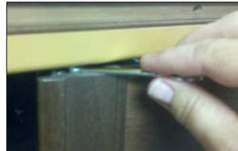
Adjustments to panel alignment are made by turning the bolt
