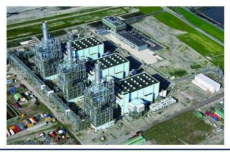
Vattenfall's Magnum power plant in the Netherlands is shown here. Mitsubishi Hitachi Power Systems (MHPS) has verified that conversion to hydrogen-fired power generation is possible on these units. Photo courtesy: MHPS
