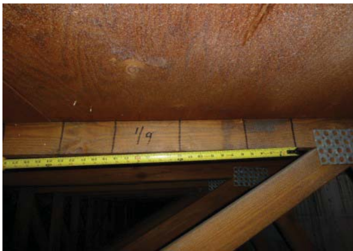
#3 ROOF DECK ATTACHMENT 6" X 6" NAIL SPACING
