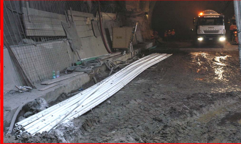
PHASE 2: Positioning pipes
