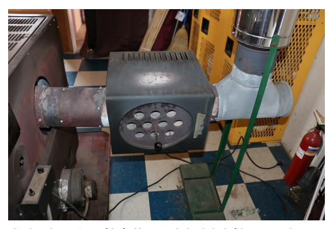
This photo shows a picture of the fan blower attached to the back of the stove. We do not use this fan and plan to eventually remove it. It constantly kicks on and off when plugged in and is annoying and ineffective.
