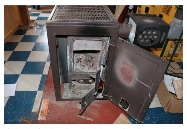
This photo shows both doors on the woodstove in the open position. The large top door is the area in which a fire is built. The smaller bottom door contains the ash pan and is used to increase decrease oxygen flow to fire in order to increase or decrease temperature.
