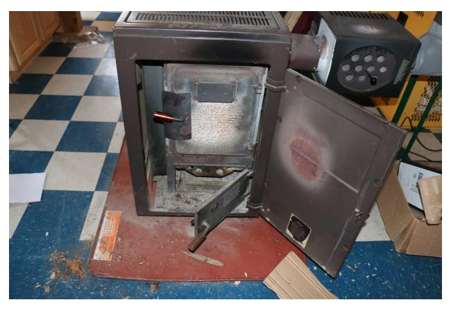
This photo shows the bottom open. This position is common when you are trying to increase heat to bring the cabin up to a comfortable temperature.
