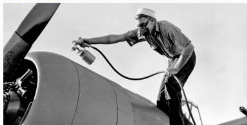
A crewman applies the Blue-Gray paint to an overall Light Gray F4F-3 aboard USS WASP, CV-7, on December 5, 1941. The directive for the Blue-Gray over Light Gray paint scheme had just been issued the previous month in November. Squadrons simply painted the Blue-Gray color on their Wildcats that were in the overall Light Gray scheme, leaving the Light Gray on the undersurfaces. Fuselage codes remained in white, and the national insignias were left as they had been on the overall Light Gray scheme. (National Archives via Bell)
