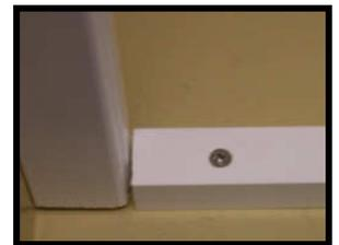
Pre-drilling is recommended to avoid splitting of the light block.
