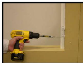
With hinge lined up, secure the bottom screw into the pre-drilled hole.
