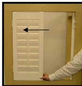
9. With all hinge pins installed, open the left panel and place the right shutter panel into the window opening and slide into position. Once panel is aligned with frame hinge, insert hinge pins into all hinges to secure the panel.
