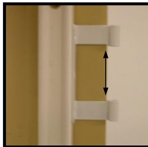
*Tip: For flush panel installation, line the backside of hinge barrel with the wall surface.*
