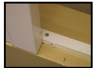
After adjustment, hold light block in place, open panel and secure the center of the light block between the magnet catch plates.
