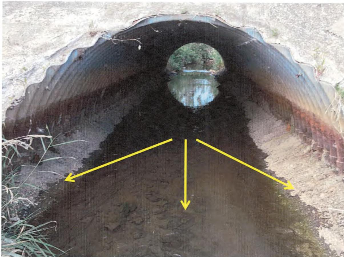
**PHOTO 1.** Sharp Rd culvert with over 2 feet of concrete and stone base along the bottom, which acts like a dam causing water to backup on Brace Property.
