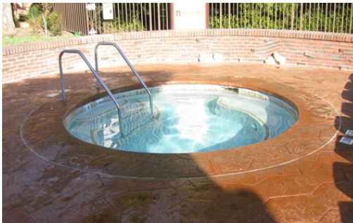
Before & After Concrete Efflorescence Removal
