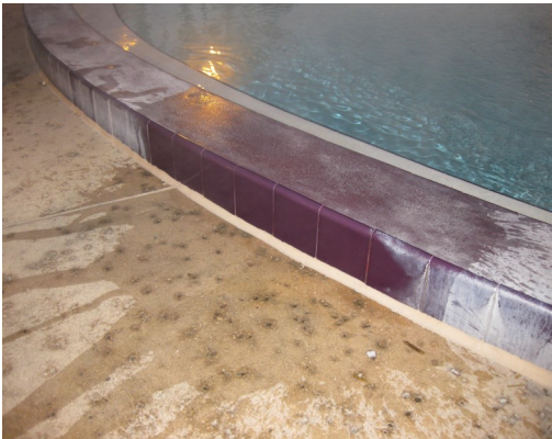
Tile & Grout Efflorescence Removal
