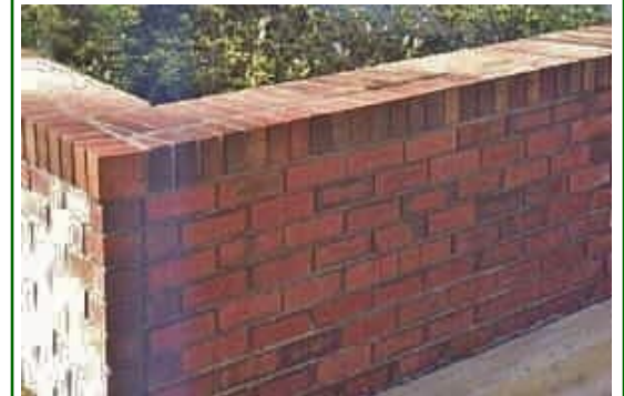
Before & After Brick Efflorescence Removal
