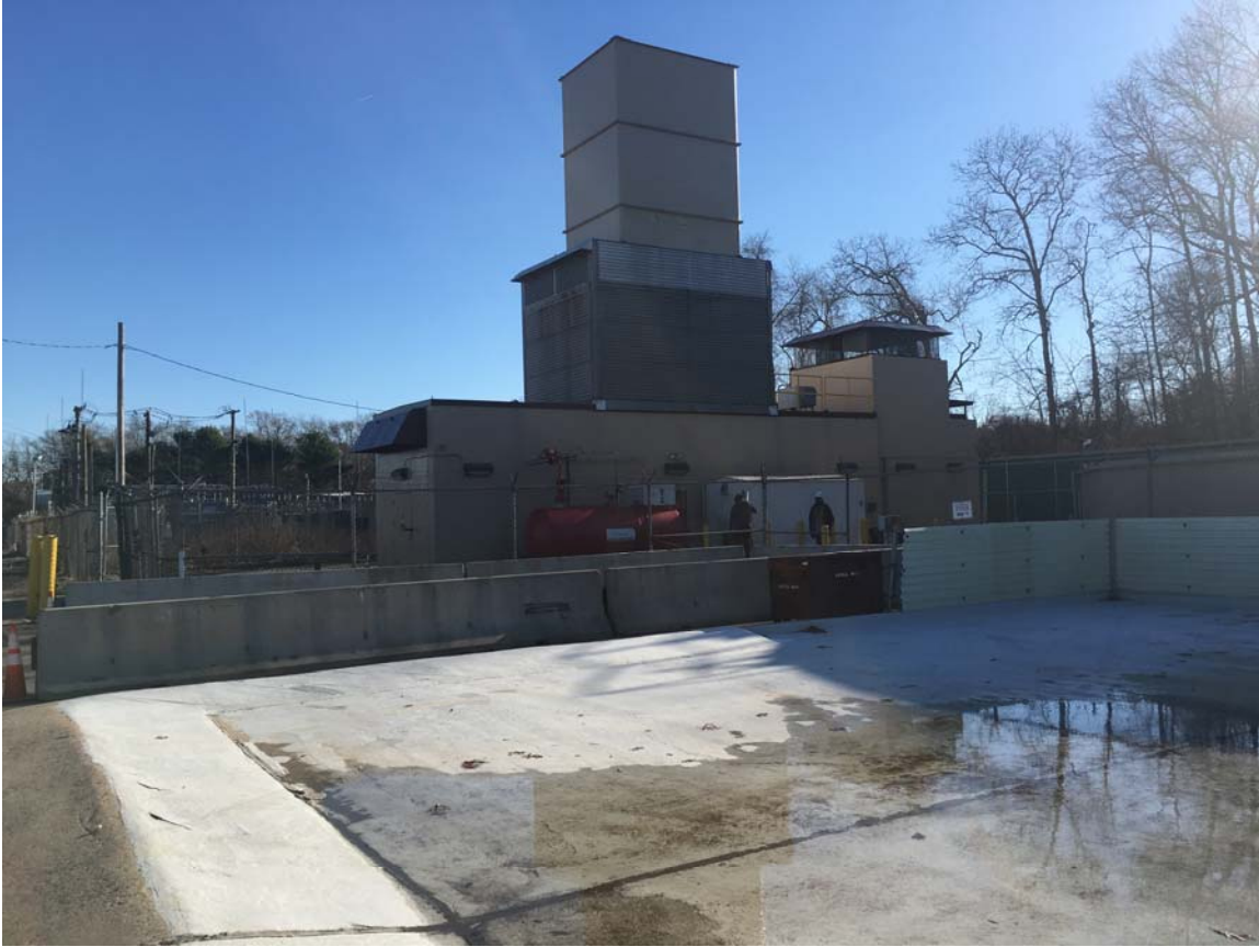
Photograph No. 1: The National Grid Generating Station located on the subject property. View is to the southwest.
