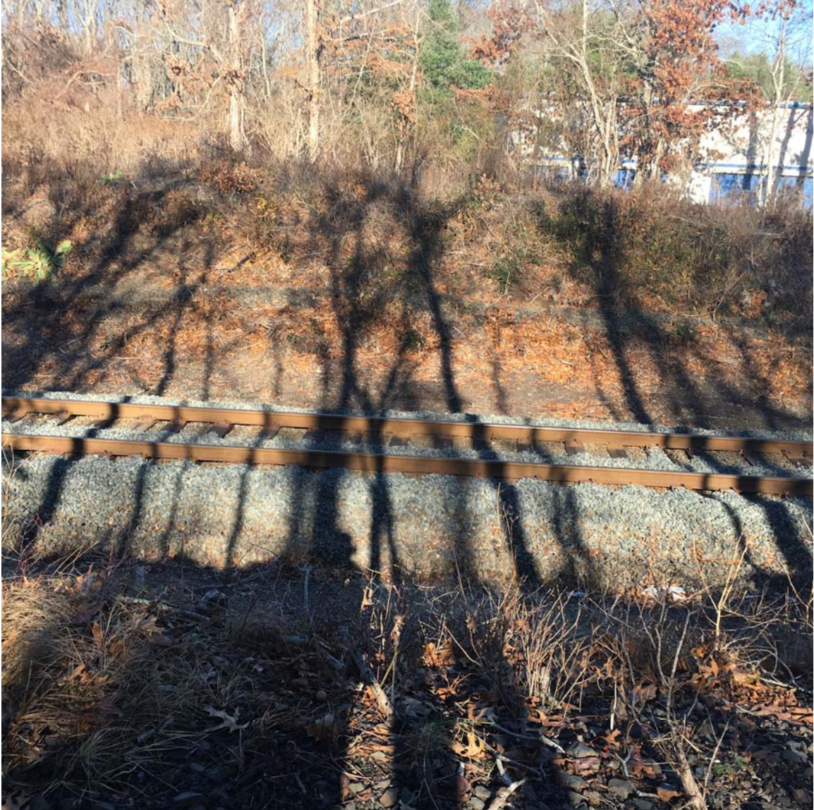
Photograph No. 3 : The LIRR right-of-way, along with a self-storage facility. View is to the north.
