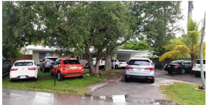
Another violation: All cars parked on the property must be on paved surfaces. There are also limits on the number of guests who may be present.
