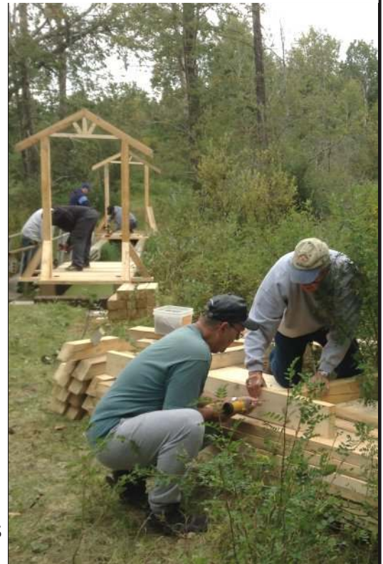
Building a bridge between Big Shell and Echo Bay
