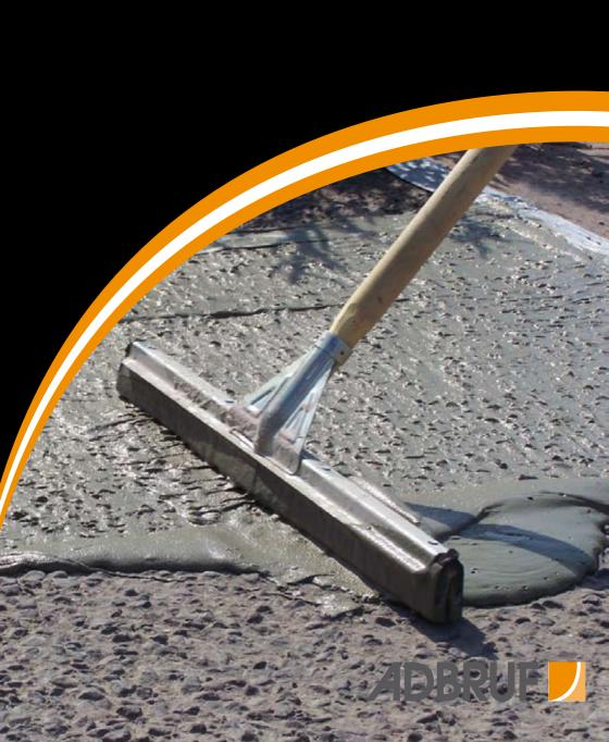
Void Filler is a polymer modified cementitious void filler and surface regulator. This system has been specially formulated to act as a strong, easily applied filler to reduce the texture and unevenness of most types of surfaces and substrates before the application of thin veneer resin surfacing type products.
