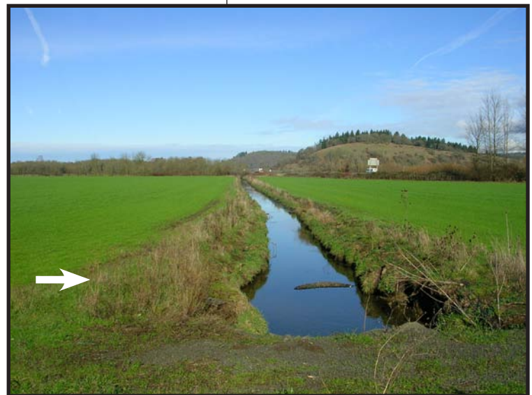
The outfall will be located in approximately this location
