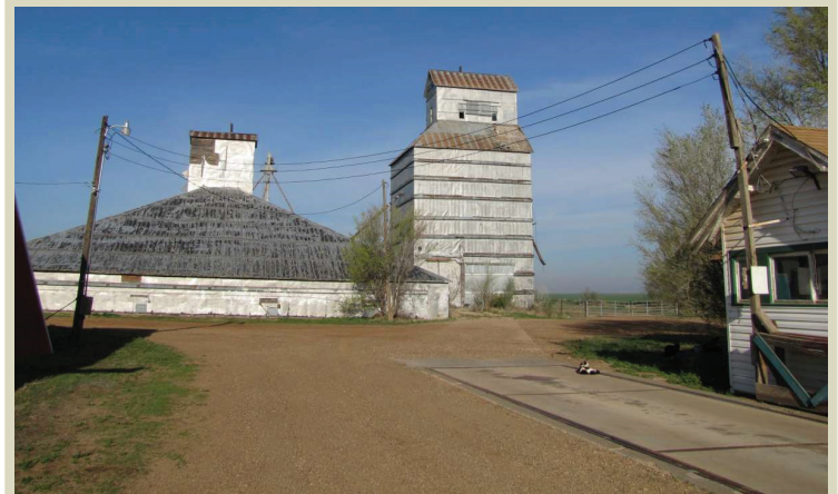
Baker Woodframe Grain Elevator, Baker (Riffe and Gilmore Company)
