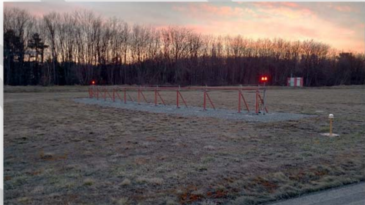
Figure 2-9 End Fire Glideslope Runway 14 End
