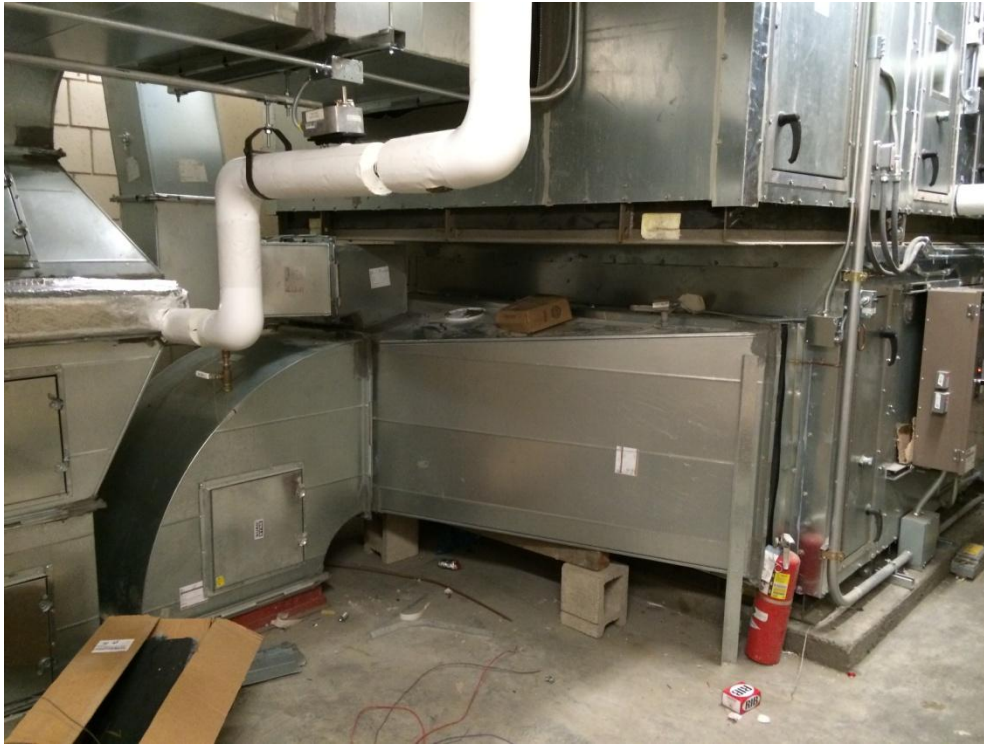
Heat Recovery AHU. Note in-duct coils and access doors for fire dampers and coil cleaning.
