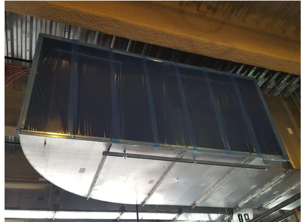
AHU Discharge, 56,000 CFM with Turning Vanes
