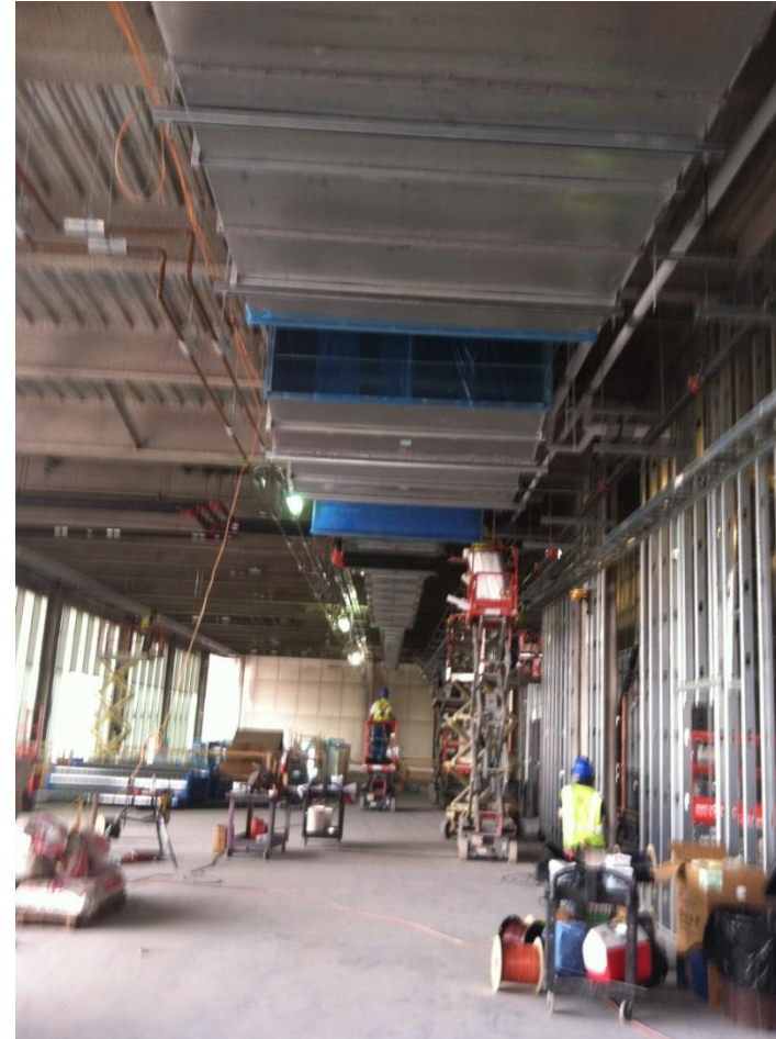
Size and height of ductwork above floor affects field labor costs by +15-20% when lifts are required.
