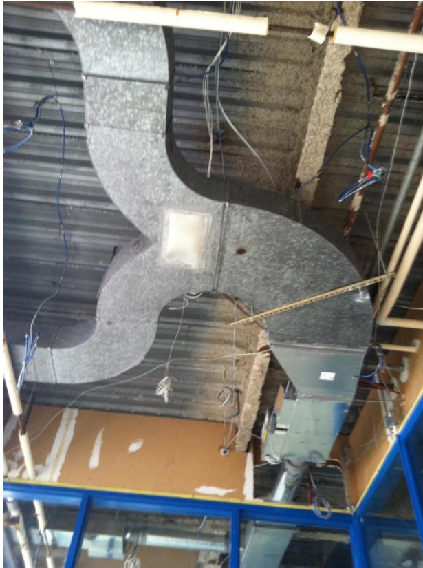
Graceful ductwork from 1977, with new terminal induction box.
