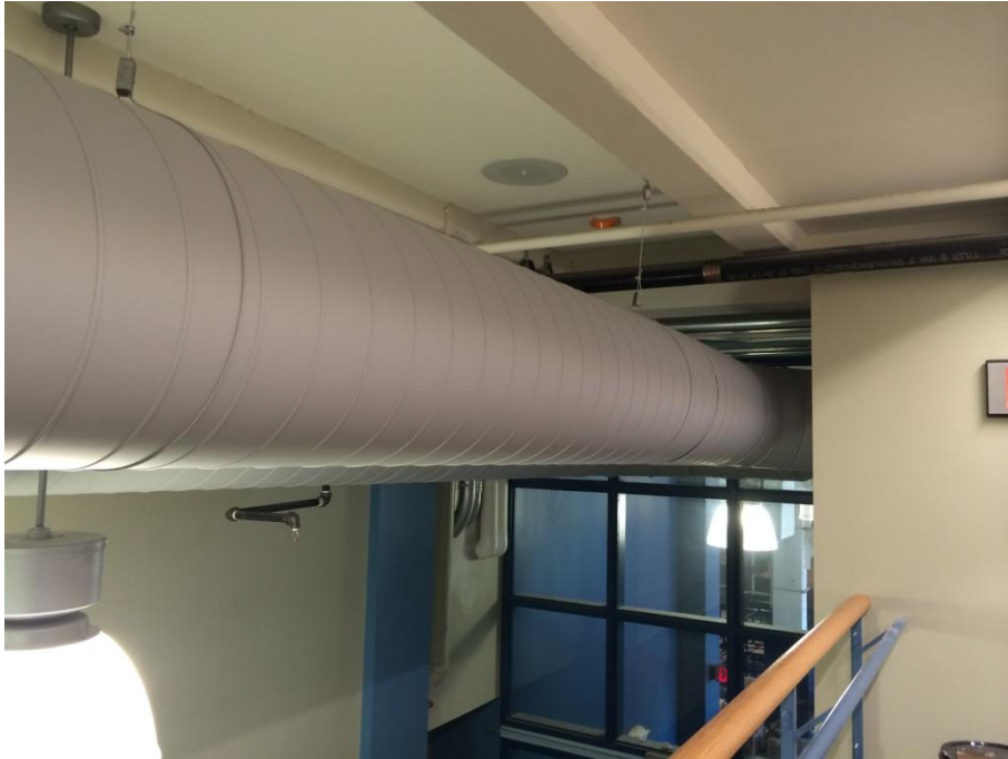
Exposed Spiral Round DW Ductwork Note “Gripple” cable hangers.
