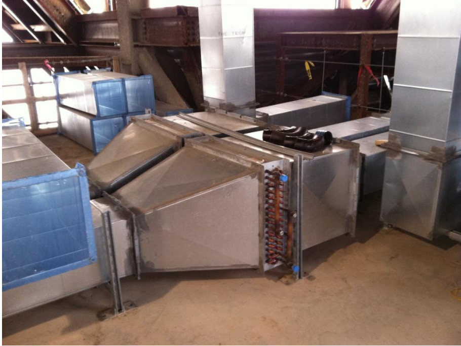
In-Duct HW Coils
