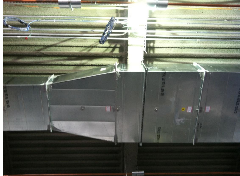
Rectangular Ductwork with Flanges and Tie-Rods
