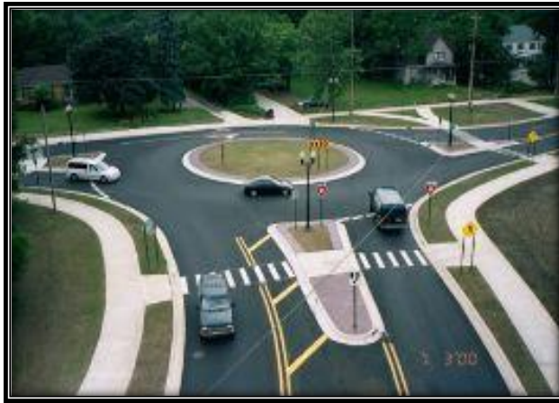
Sample Design of Three-way Roundabouts
