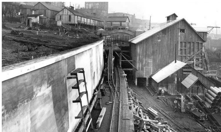
Above: Archival photos of early tunnel construction
