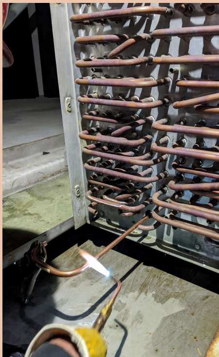
Return Bend Replacement
