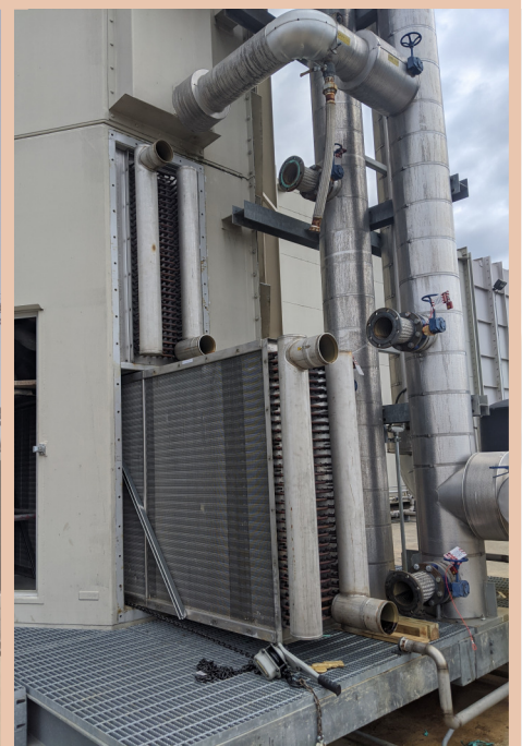
Safe Module Removal
