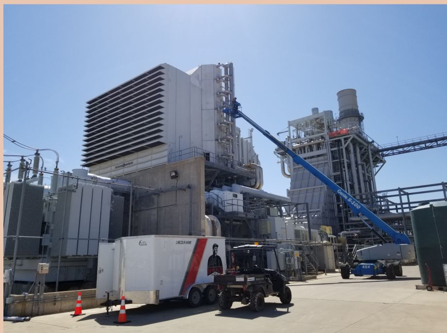
Complete Turn-Key Chiller Repair & Cleaning
