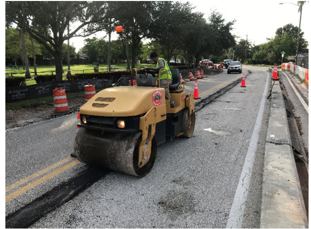
The rutting in the center of the road gets repaired
