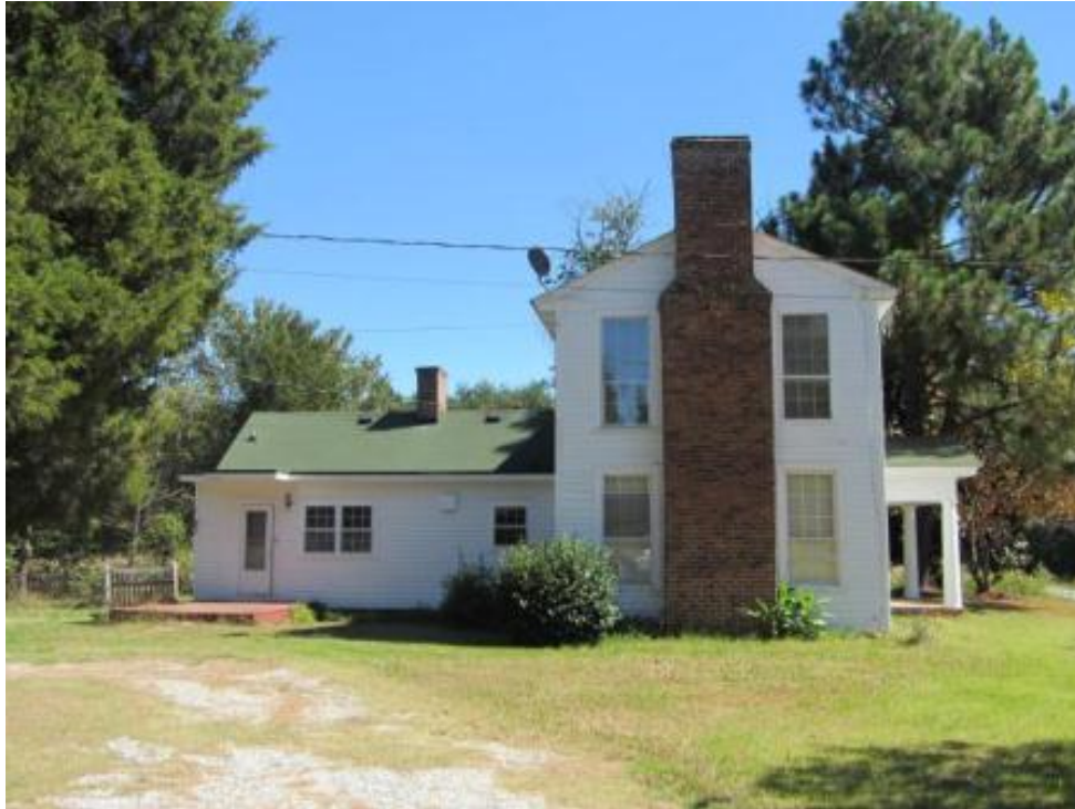
Figure 17. NCDOT Survey #45, Dr. Joseph A. McLean House (GF-1535), 6069 Burlington Road, Guilford County, looking east; main house and entrance portico are on the right and the rear ell with the west addition is on the left.
