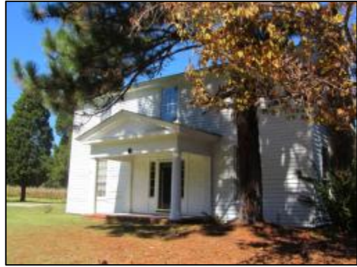
NCDOT Survey #45, Dr. Joseph A. McLean House (GF-1535), looking northeast.
