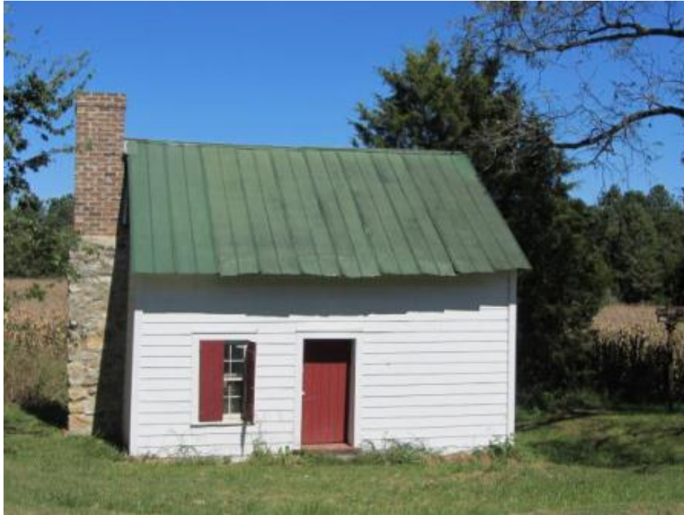
Figure 19. NCDOT Survey #45, Dr. Joseph A. McLean House (GF-1535), 6069 Burlington Road, Guilford County, log kitchen, south façade, looking north.
