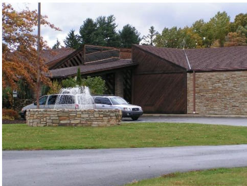
Main Building. Check in here.
