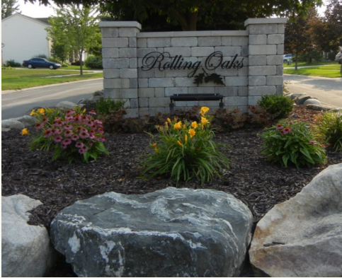
Entrance renovation complete in 2011
