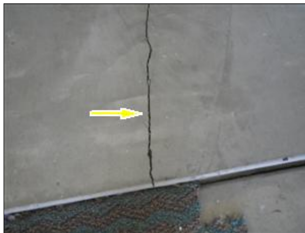
cracking
