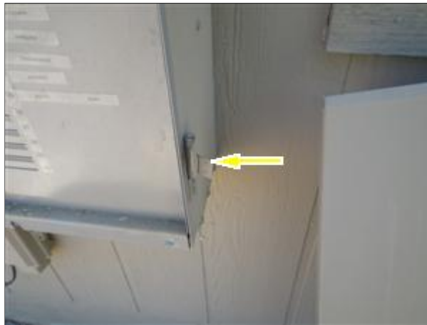
broken hinge
