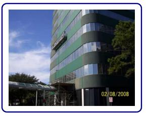
North Loop Center I is is a twelve-story office tower located at 1235 North Loop West in Houston, Texas. The structural steel framed building was constructed around 1981. The exterior walls are constructed with an exterior insulation finish system
