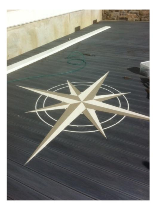
Install inlay in the same position as your tracing and secure with color matched screws or Cortex screws and plugs
