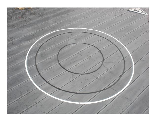
Using a router with a circle cutting jig, cut circles in deck 5/16" deep and install azek trim into grooves. Use PVC glue to secure circles. Place your joints in the area that will be cut out for the inlay.
