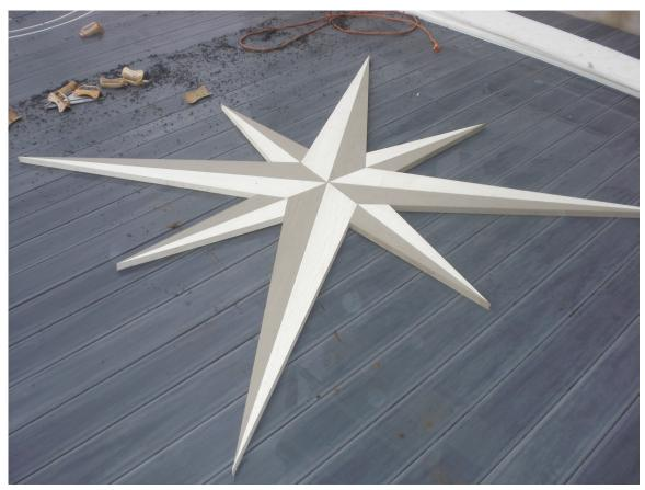
Turn your inlay over and place it on the deck where the blocking has already been installed under decking and trace the location
