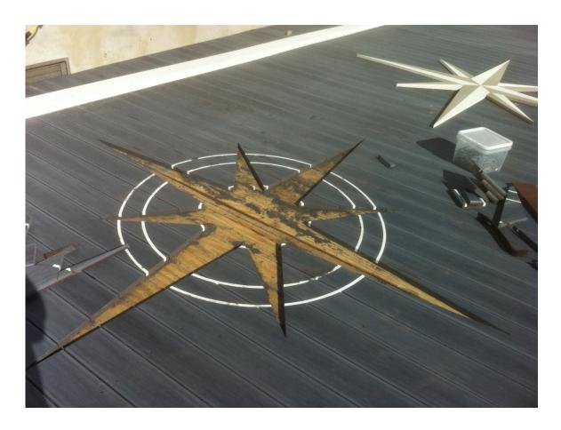
Cut out inlay along traced lines, note solid blocking under inlay, be sure to drill holes tin blocking to insure drainage
