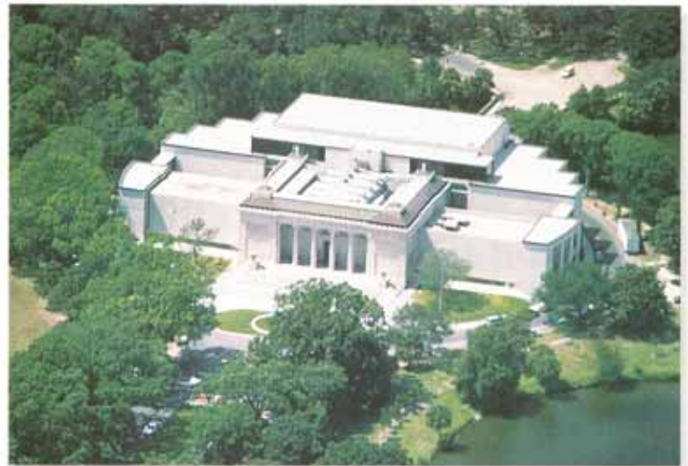
The New Orleans Museum of Art roof features Zonolite Insulating Concrete and Paradiene 20/30 SBS modified bitumen. (PHOTO COURTESY OF SIFLAST, IRVING, TX.)
