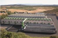
Waste air exhausted from the biotunnel is mixed with air coming from the hall (always maintained in slightly **negative pressure conditions**) and processed in a centralized odor control system, typically consisting of one or more blowers, an air humidifier and a biofilter.
