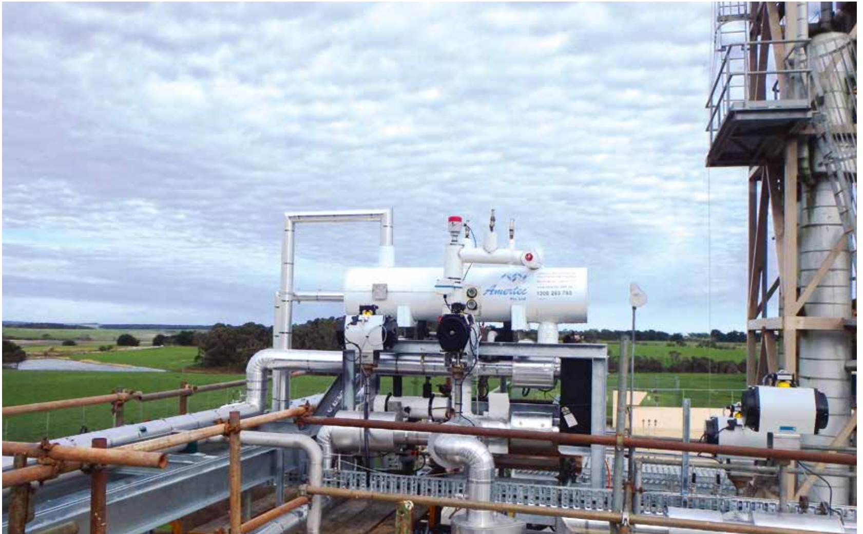
BOC's Boggy Creek facility is home to a unique flooded CO 2 cascade system.
