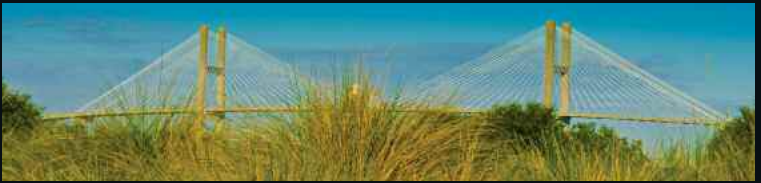
Talmadge Memorial Bridge Gateway from Savannah to South Carolina***
