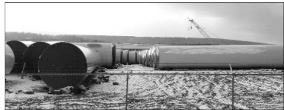
A field of main support sections for large wind generators.
