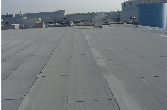
Photo credit: Structural Research, Inc.
