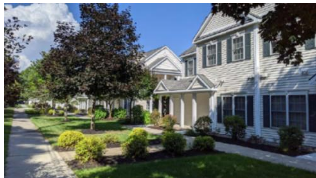
Figure 7. This multifamily development includes many design features consistent with the TC Design Standards including setbacks, sidewalks, front yard landscaping, traditional building styles, two story buildings, facade breaks, and traditional windows.
