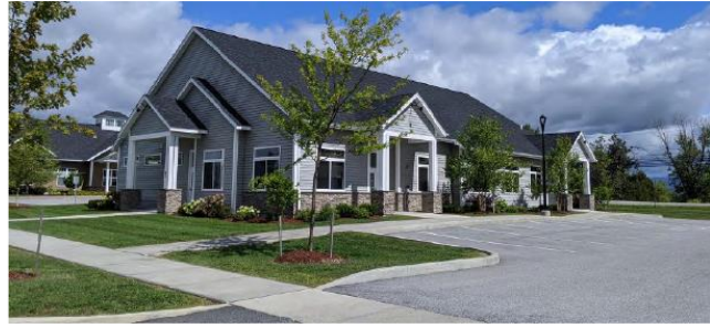
Figure 1. Example of a building with an appropriate front facade and the main entrance on the side with a side-oriented parking lot
