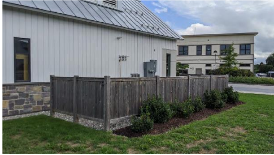
Figure 12. This example shows an effective use of landscaping and fencing to screen utilities.
