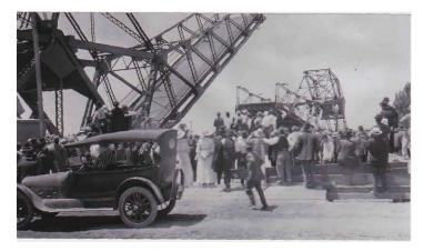
The deck was wooden and became heavy when sodden with rainwater. To counterbalance this weight, extra concrete blocks were seasonably added to the huge concrete counterweights. A sidewalk on the downstream side was added after several vehicle-pedestrian accidents occurred on the bridge. Funds to add the walkway were raised by the Delta Progress Club and the Walnut Grove Boy Scouts.
