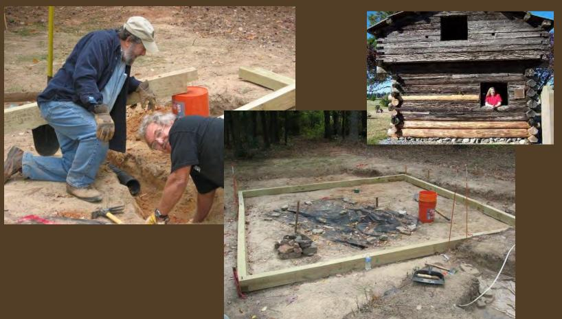
Installation of drainage system and 4x6 beam outline of Blockhouse footprint.
