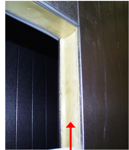
Exposed insulation – must be sealed or closed, depending on the zone
