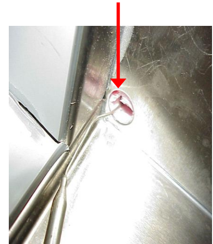
Exposed insulation – must be sealed or closed, depending on the zone
