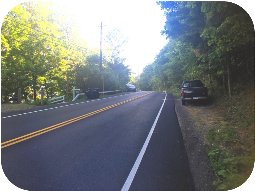
Picture looking South on W. Lake Rd. Parking is on the right where the green truck is parked. Keuka Villa is across the road on the left. 52 feet of end to end parking.
