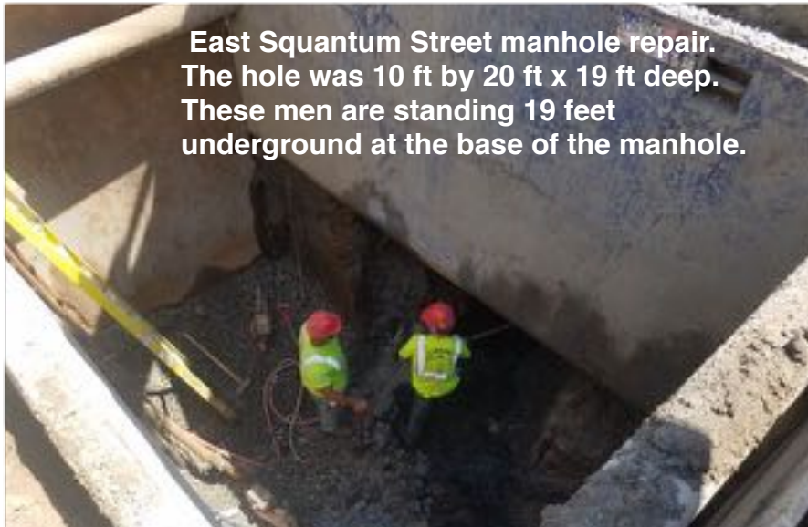
Getting ready to drop the manhole in place
