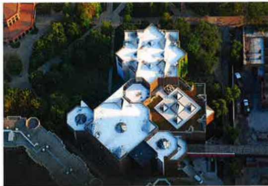
Reflective roofs, ballasted and garden/vegetative roofs meet Chicago's 2009 Energy Code.
