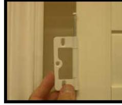
Completely install the hinge pin.
