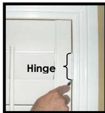
Mark should be made on the wall/jamb at the bottom of the hinge.
