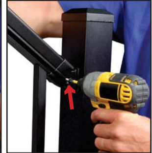
(b) Anchor Bracket w/ pivot screw
