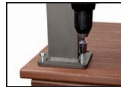
Fasten Post to Deck Surface
