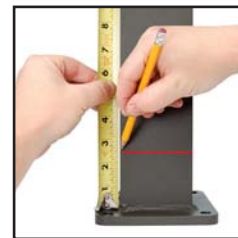
Measure up 2-3/8" from top of base plate
