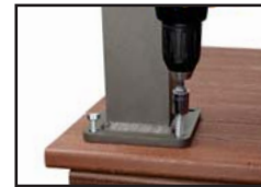
Fasten Post to Deck Surface
