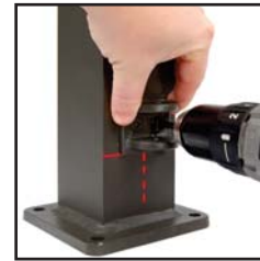
Center and fasten backer plate to post with centered pivot hole on bottom
