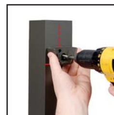
Center bracket and attach to post
