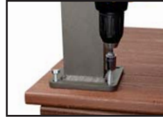
Fasten Post to Deck Surface
